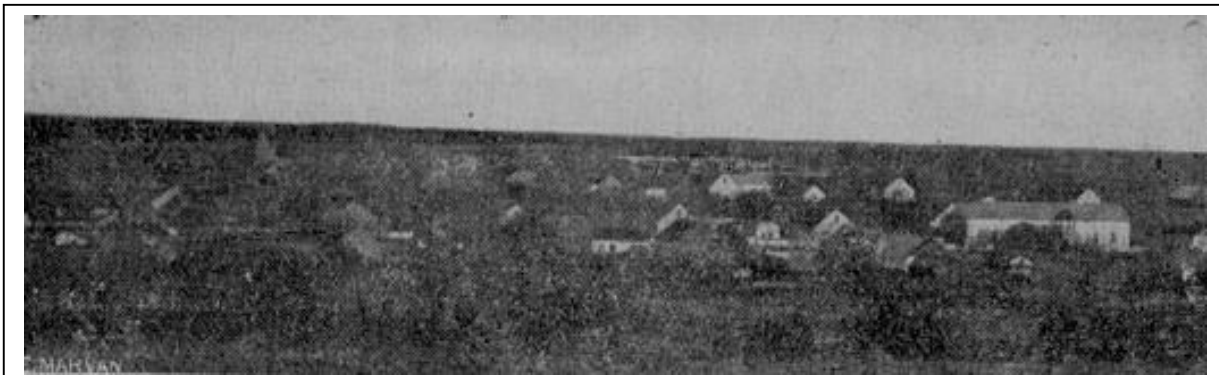
Overall view of Mannsburg
