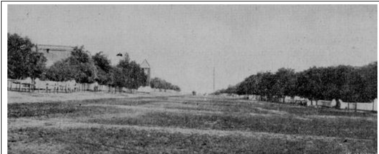
Street view of Mannsburg
