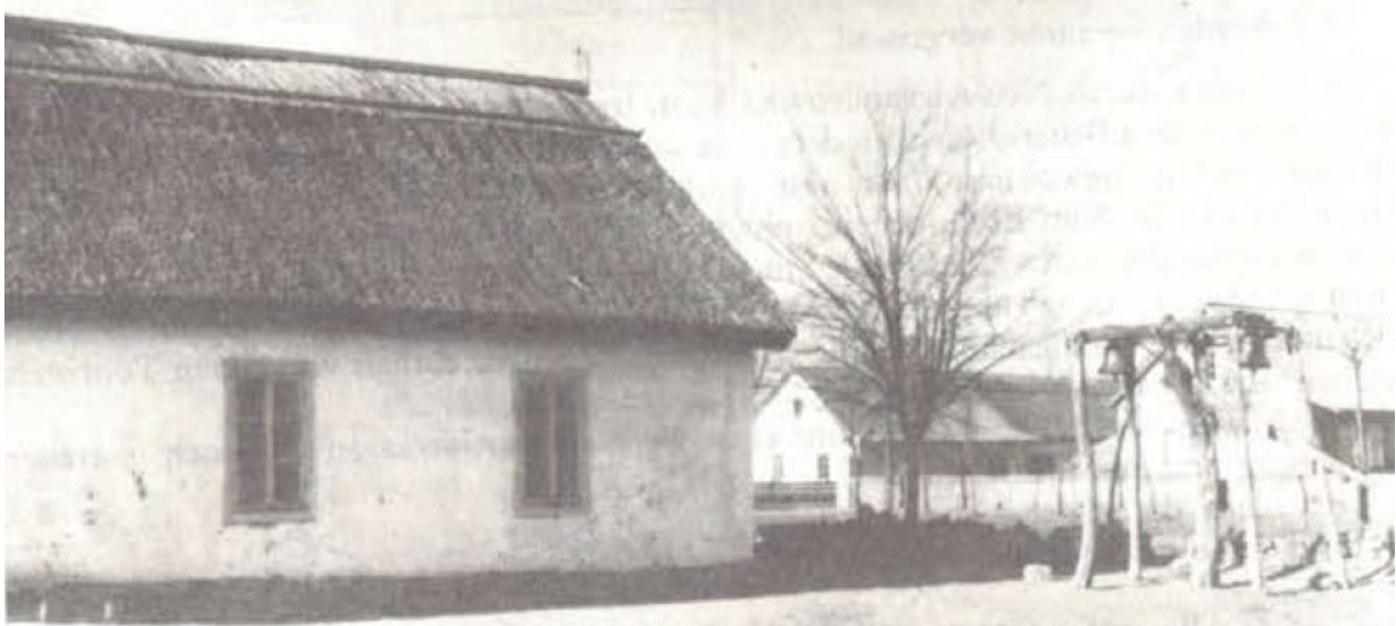
Parapara 1940. Old School with Bell Tower
